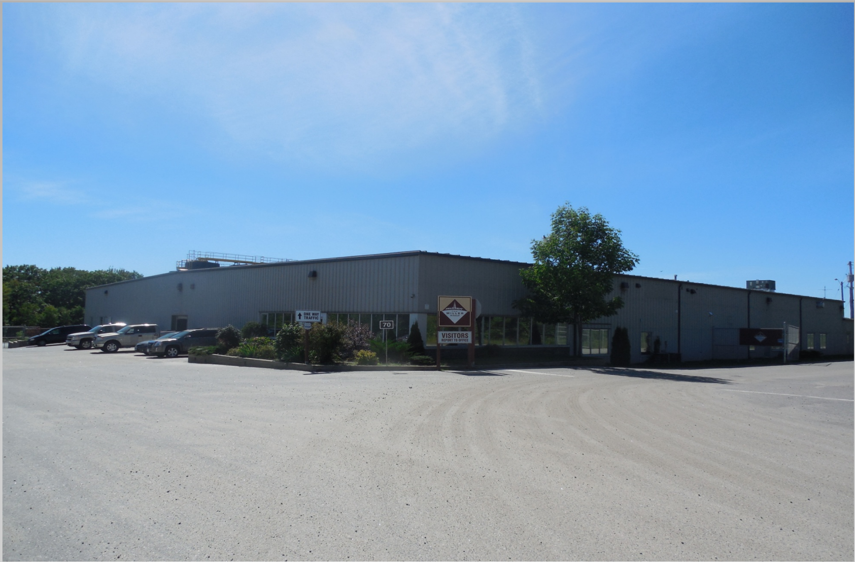
Lessee Miller Paving Ltd, McAsphalt.
