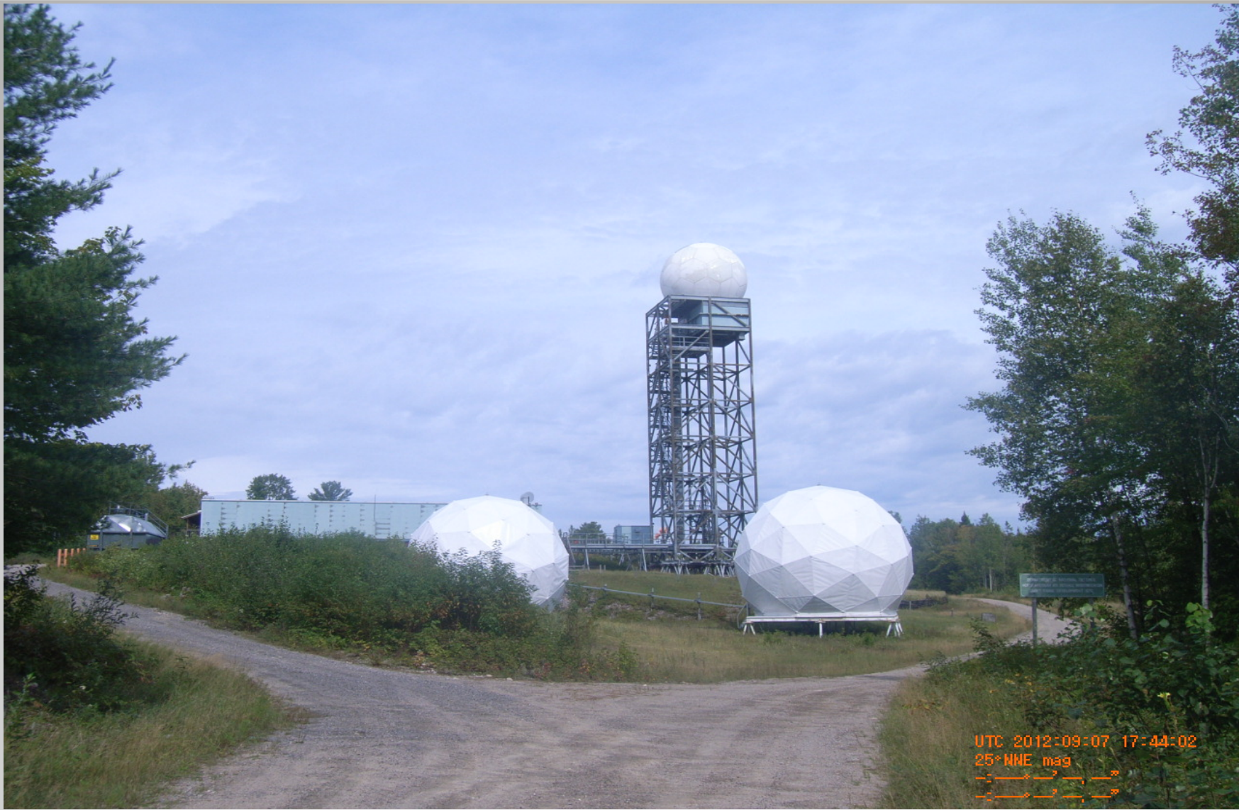
Short Radar Range Base-NavCan Lessee
