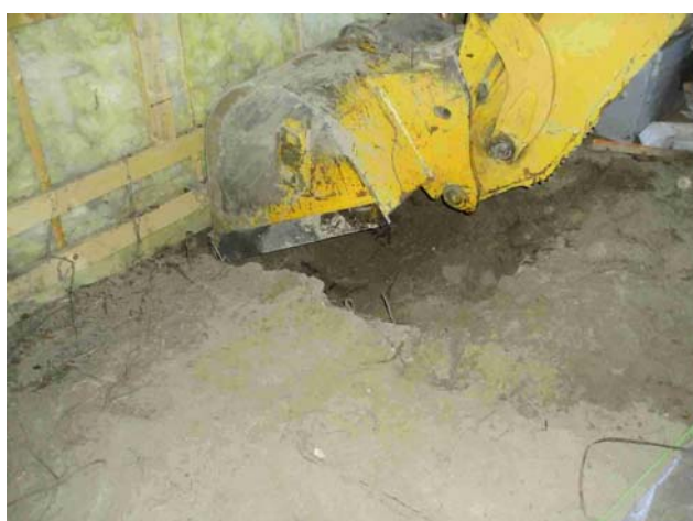
Photograph 13: Excavation of Impacted Soil from Agriculture Shed.
