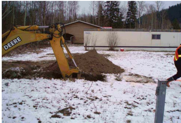
Photograph 12: Test Pit Excavation.
