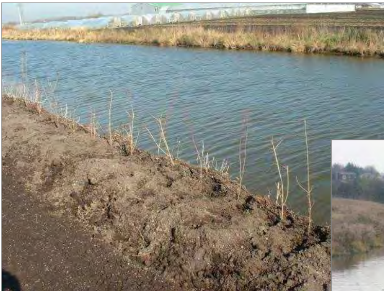
Figure 3-11: Riparian plantings undertaken in agricultural areas to mitigate bank erosion and prevent nutrients and sediment from reaching the watercourse
