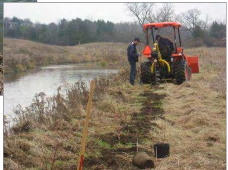
Figure 3-11: Riparian plantings undertaken in agricultural areas to mitigate bank erosion and prevent nutrients and sediment from reaching the watercourse
