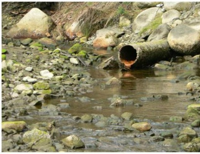
Photo: Storm drain discharging unknown material on the shoreline of a Squamish Nation reserve. Used by permission: Westland Resource Group
