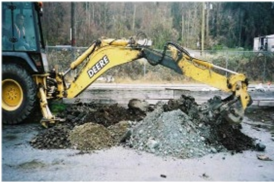
Photo: Squamish Nation Environmental Site Assessment Test Pitting. Used with permission: Squamish Nation, B.C.
