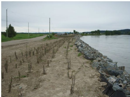
Photo: Riverbank erosion protection project – post construction remediation and fish habitat enhancement. Used with permission: Lheidli T'enneh.
