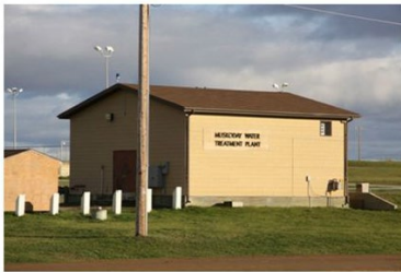
Photo: Muskoday First Nation Water Treatment Plant, Saskatchewan. Used by permission: Muskoday First Nation
